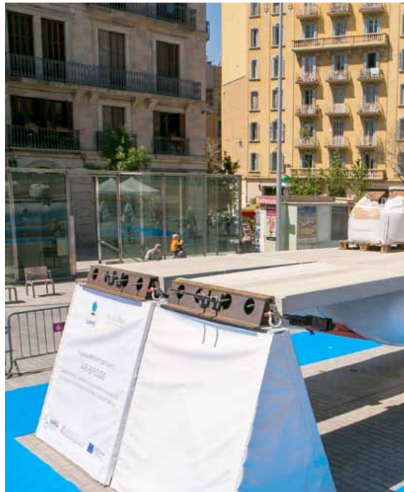
Buildair's lightweight bridges with pneumatic beams that can be installed quickly in the event of an emergency.
